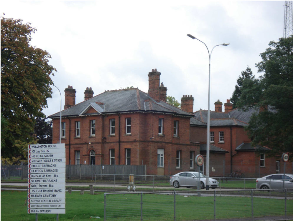
Alison House, Queens Avenue, Farnborough – north elevation, setting and relationship to adjacent (and mirrored) Cranbrook House (to the south)
