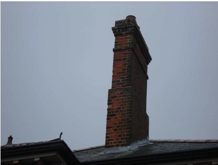
Alison House, Queens Avenue, Farnborough – Chimney detail
