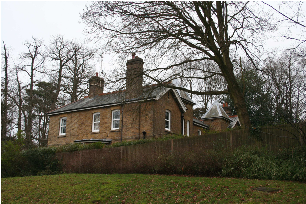
Badajos Lodge, Knollys Road, Aldershot –south and west elevation
