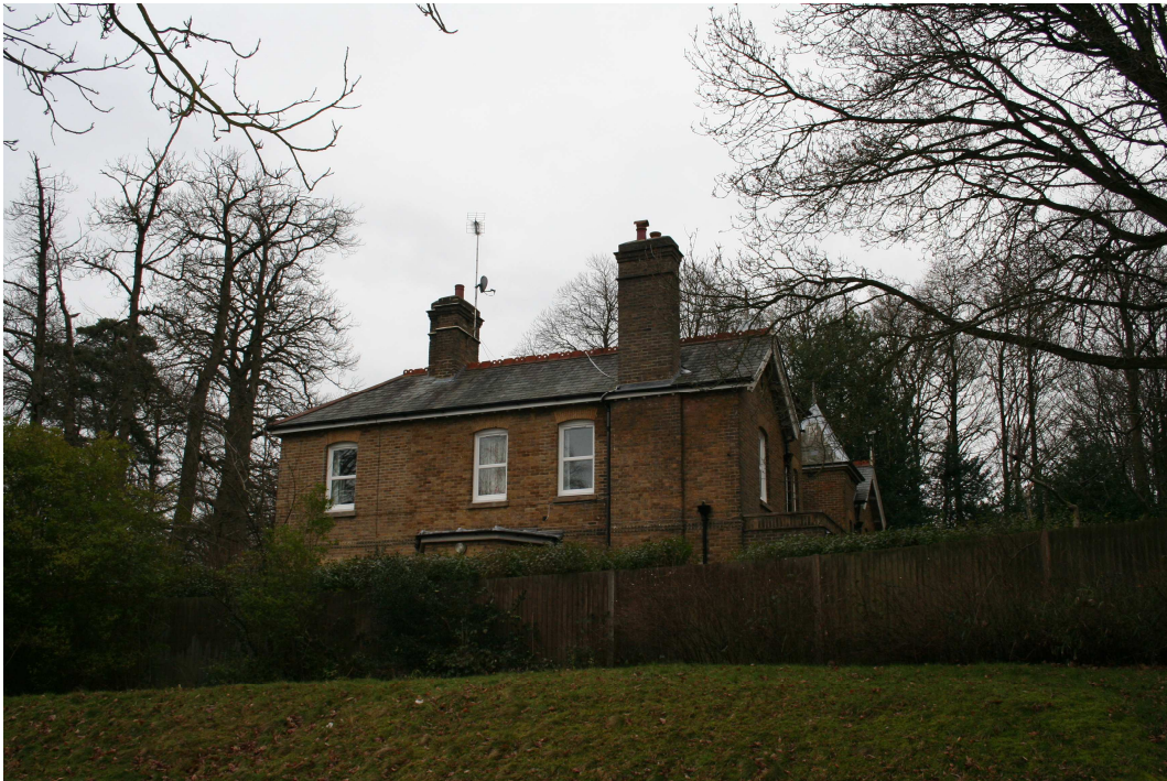
Badajos Lodge, Knollys Road, Aldershot – west elevation
