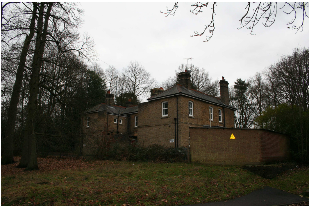
Badajos (foreground) and Salamanca (background) Lodges, Knollys Road, Aldershot – north elevation
